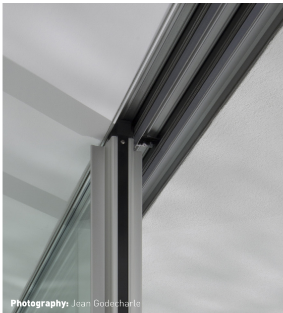
View of the open pane, showing upper frame built into the false ceiling.
