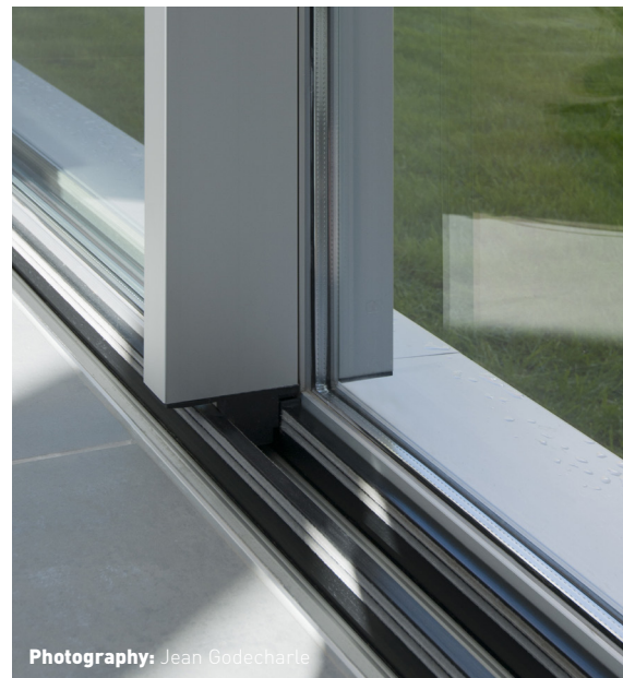
Detail of the central overlap of two panes, showing lower frame flush with the outer and inner pavement. The depth of the pane upright depends on the pressure it must support so that the glass does not exceed its stress threshold.
